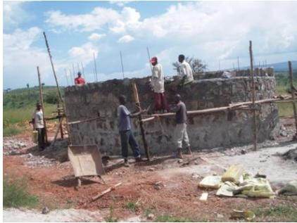
to build a 300,000 liter community cistern in Chonyoyo, adjacent to a storage building with a large roof and gutters to fill it. They also installed a solar powered pump. Student groups, in addition to helping to provide funds for the project, were put to work tutoring,
